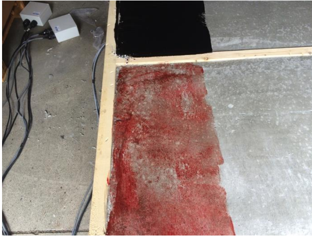
Figure 3 Application of Primer to Concrete Slabs on Day 1
